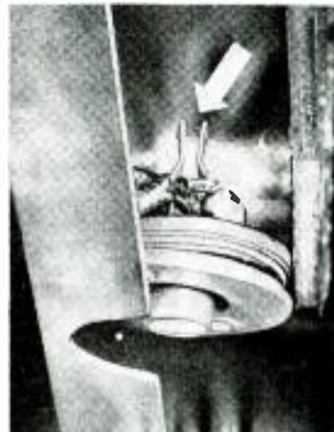
One of the Pittsburgh BBB's faulty circuits.
